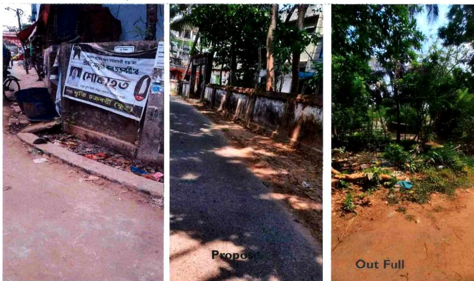
D3-B: Construction of RCC Drain Starting From Hazi para Md kutub Uddin Shaheb Mosque to Kashkhali Canal ch 0.00m-408.00m, Under Raozan Pourashava.
